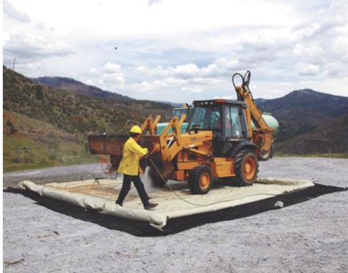
Figure 1. Flexible mat type of vehicle wheel wash, from <http://www.fs.fed.us/eng/pubs/pdf/05511203.pdf>
